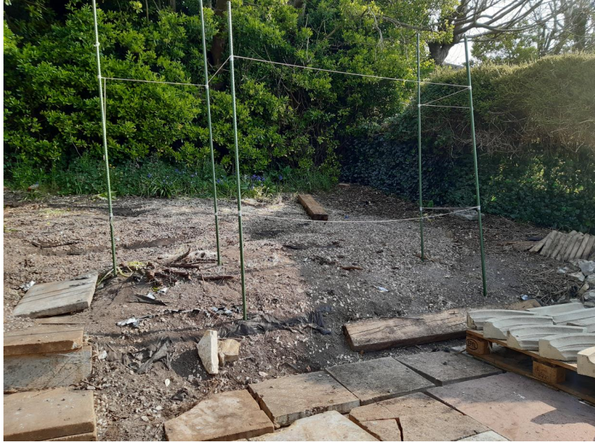
Area of proposed folly with mock up showing the level of the raised platform (lower string) and the top of the structure (higher string).
